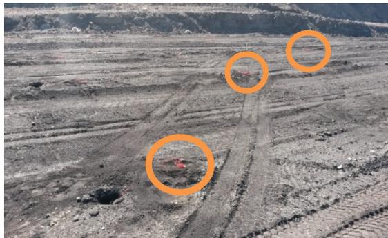
**Image 2. Watertruck tracks over unloaded hole and close to detonators**
